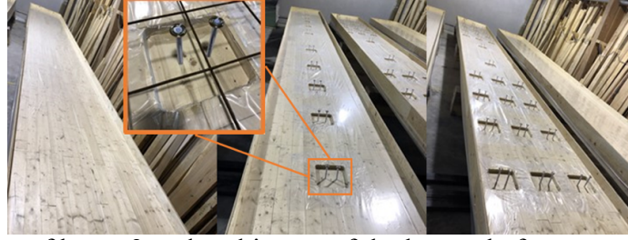
Fig. 1: Plan of beam 3 and real image of the beams before concrete casting
