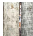
Fig. 12: fungi colonization on the cladding at the craft laboratory, photo by the author.
