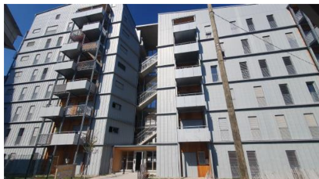
Fig. 1 : The “Haut-Bois”, R+8 (left), concrete stairwell (middle), R+5 (right)
